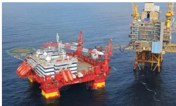
Floatel Superior alongside Oseberg, West coast Norway
